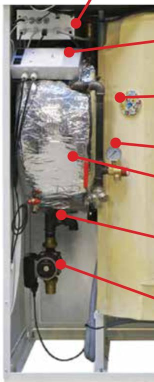
Supplementary electrical heating of 2 x 3 kW Ensures indoor heating during periods of severe frost.
